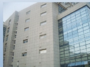
PROJECT IN UAE, Wall cladding Material--- G554 Flamed + Brushed. Flooring---G681 polished and Rajp Alicante
